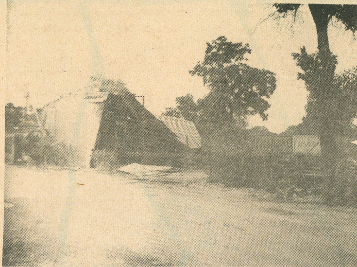
Going, going, almost gone. The old Farmhouse building in Houston is shown with only a partial skeleton remaining — the result of two fires and a demolition company. The owners, meanwhile, are showing off their new location at 2710 Albany.
