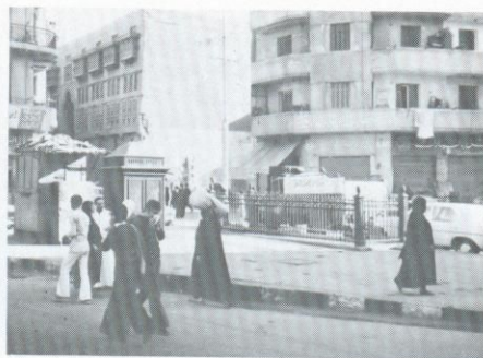
Underground John on Al Azhar St.
